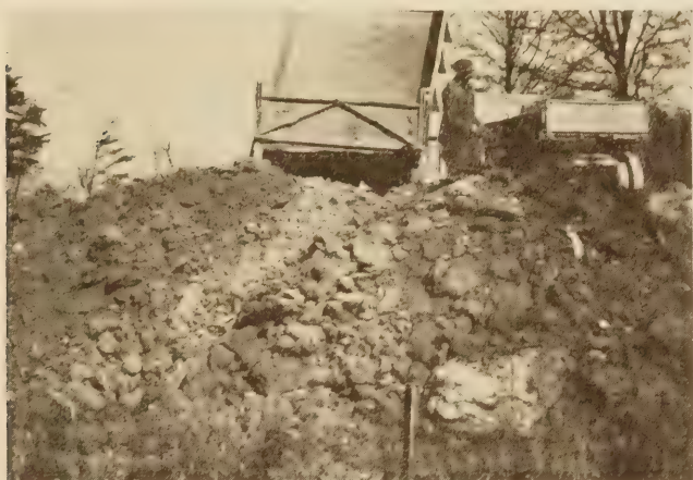
FIGURE 16.—FILL BEING CONSTRUCTED OF MATERIAL CONSISTING OF CLODS
